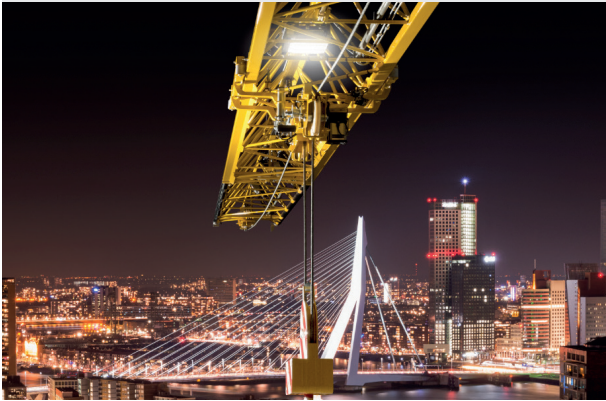
Four LED floodlights are mounted in the jib and tower.
