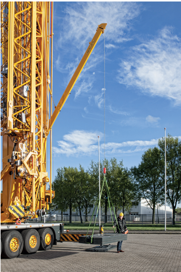
Auxiliary crane for placing the steel pads
